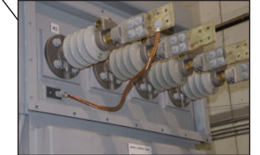
Side Mounted LV Bushings
