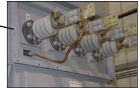
Side-Mounted LV Bushings
