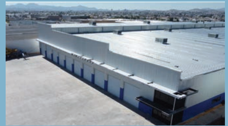
VTCW - P2, second plant built in 2022
