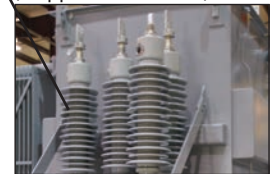
HV Bushings & Arrestors (Shipped demounted)
