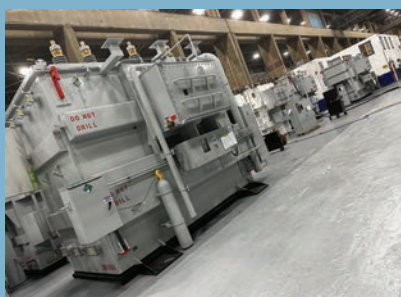
Pocatello plant floor
