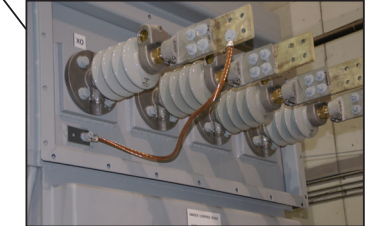
Side Mounted LV Bushings
